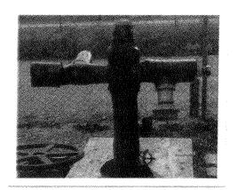
Well casing vents, and air relief valves raised 3' above grade surface.
